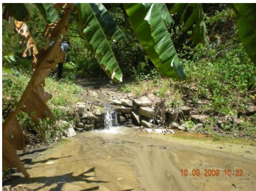
Figure 4 - Silted-up dam overflow in a sub-humid area of Pesqueiro River Basin in Aratuba-CE.
