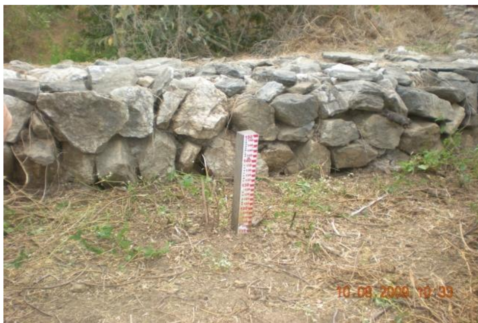
Figure 5 – Dam silted up by more than 1.10 m over the period of 8 years in Cangati River dry area in Canindé-CE.
