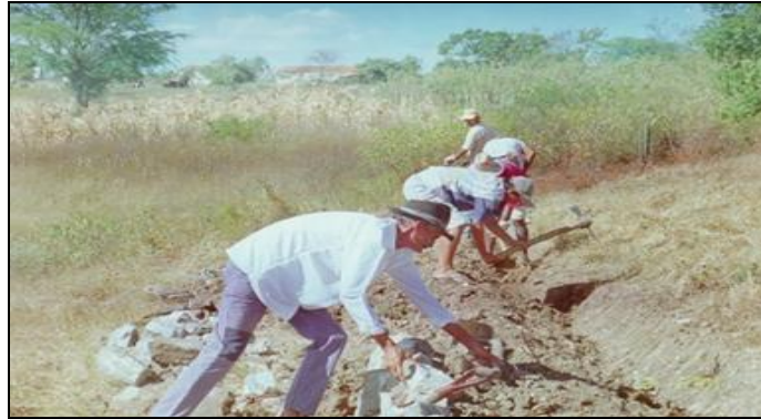
Figure 4 – Iguaçu farmers constructing a stone barrier
