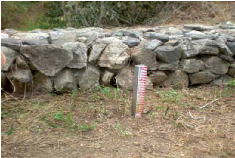
Photo 6 - Stone Dam – Zero Base Technology (TBZs)
