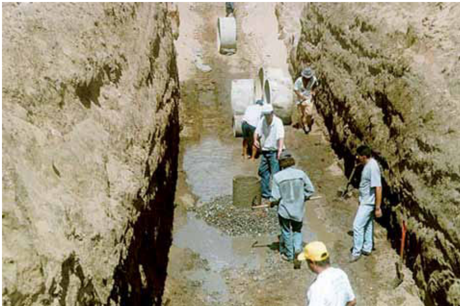
Photo 9 –Canvas Disposition in an Underground Dam
