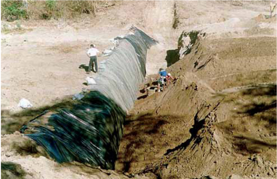
Photo 10 – Aspect of the Trench of an Underground Dam, Showing in the Center, the Piezometric Well Foundation Source: João Bosco de Oliveira.
