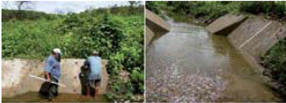
Photo 2.08 – Installation of limnimetric ruler in flume 02
