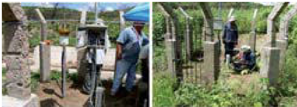
Photo 2.06 – DCP installation in flume 02, data collection and evaluation of equipment calibration.
