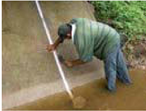
Photo 2.07 – Installation of limnimetric ruler in flume 01
