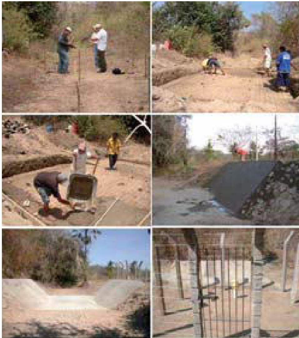
Photo 2.03 – Construction stages of flume 01: plotting, iron structure, concrete application, finish and completion.
