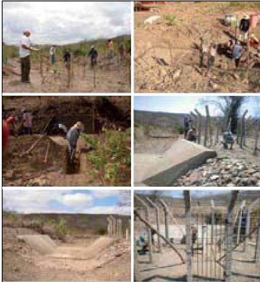
Photo 2.04 – Construction stages of flume 02: plotting, iron structure, concrete application,, finish and completion.
