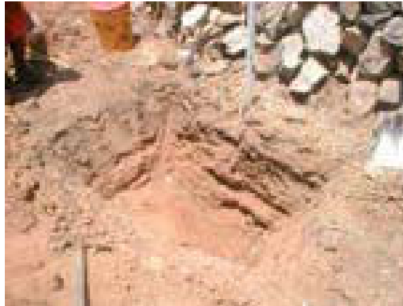
Photo 3.08 – Trench for ruler installation in successive dam
