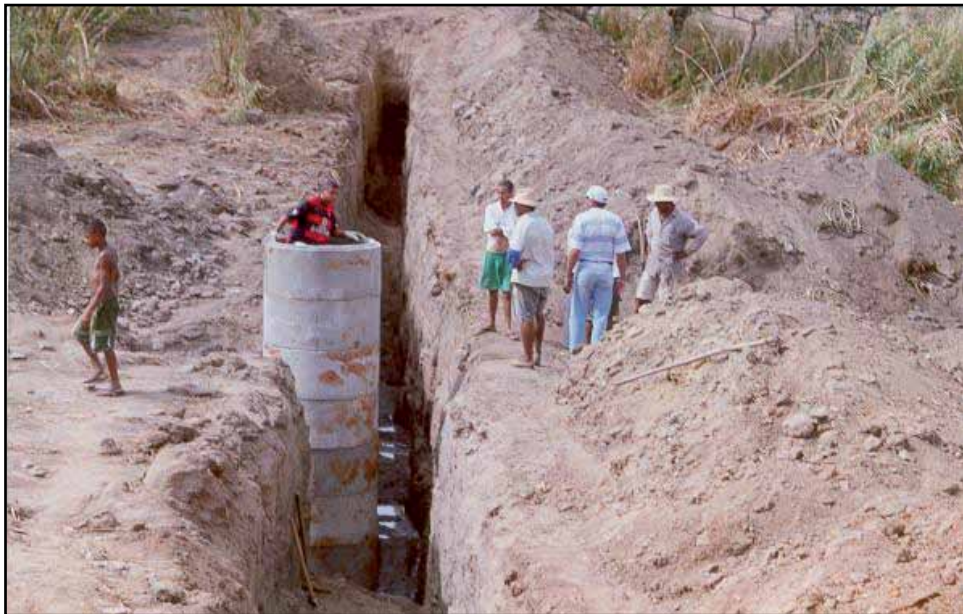
Photo 6 - Aspect of an Underground Dam under Construction
